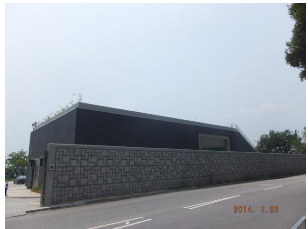
Photo 2 – The built boundary wall along the western boundary of Area A.
