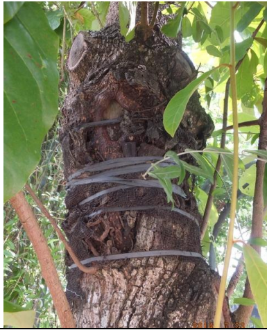
Photo 25 – The trunk of the transplanted tree U53 was still tied tightly by strings and hessian wrapping.
