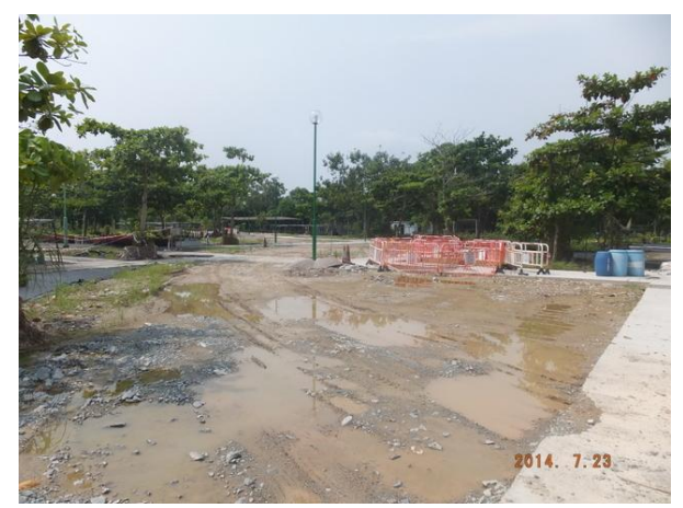
Photo 6 – Phase 1 works area was still demarcated with loosed barrier tapes.
