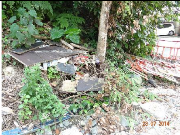
Photo 25 – Excavated soil and rocks, and construction materials were noted piling close to the trunk base of the retained tree T103.
