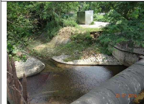
Photo 17 – No direct water discharge into the upper stream of Wai Ha River was observed as the construction works have been concentrated at the lower end of the river.
