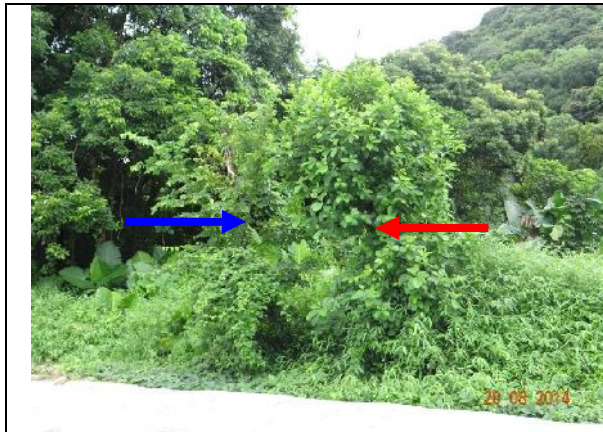
Photo 19 – Topped trees T167 (Red arrow) and T168 (Blue arrow) were in poor health condition with vigorous development of epicormics. Excavated soil was noted piling around the trunk flare.
