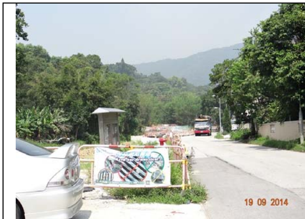
Photo 1 – Temporary hoardings have been erected along Tung Tsz Road opposite to Wai Ha.
