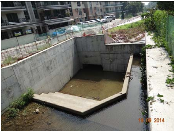
Photo 3 – Construction works have been stopped next to Wai Ha River.
