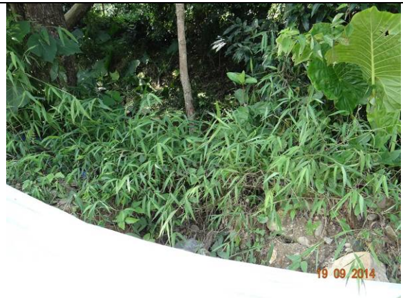
Photo 28 – Excavation work was noted previously between T153 and T155 in April 2014, and exposed roots were noted on these two trees. Surrounding ground was covered by vegetation.
