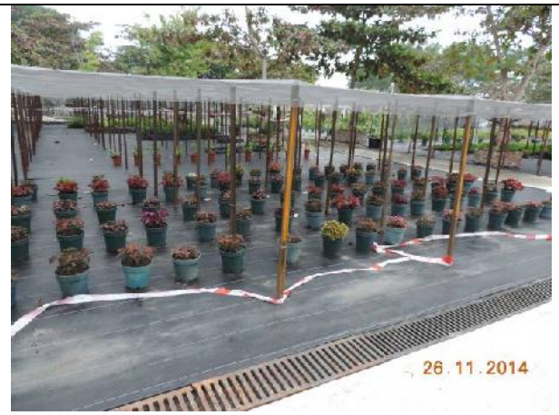
Photo 8 –Installation of shelters for potted plants was almost finished.
