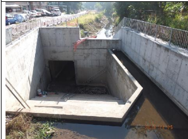
Photo 3 – No active construction works was carried out in the built box culvert and its associated structure.
