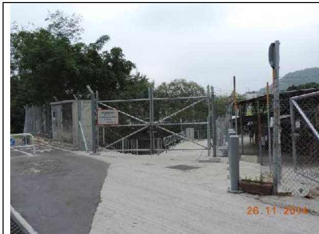
Photo 1 – Temporary construction hoardings have been removed around the works area at Wai Ha River estuary and a new gate and chain-link fence were erected to demarcate the area.
