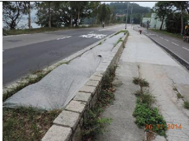
Photo 3 – The roadside planters along Ting Kok Road were hydroseeded and shrubs were planted in the planters.
