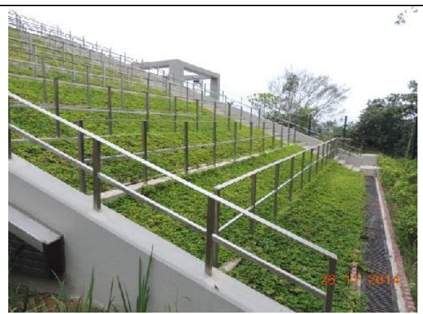
Photo 12 –The ground cover was replanted on the sloping green roof in early August 2014 and it was in fair condition.
