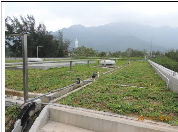
Photo 13 –The green roof was vegetated with ground cover Arachis duranensis .
