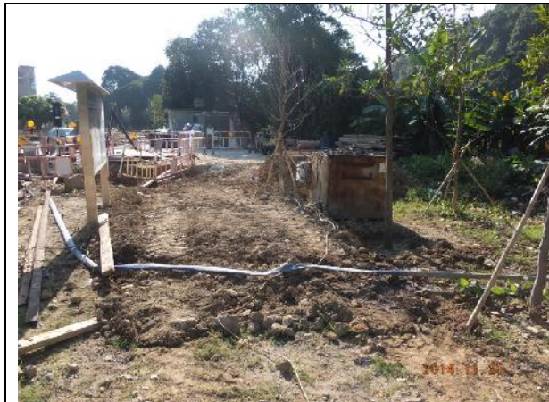
Photo 7 – Minor civil work was conducted for building a refuse collection point opposite to Wai Ha area.
