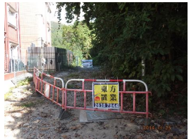
Photo 12 – Construction works have been stopped at the end of the Treasure Spot Garden II near the retained tree T103 and it was surrounded by temporary construction barriers.
