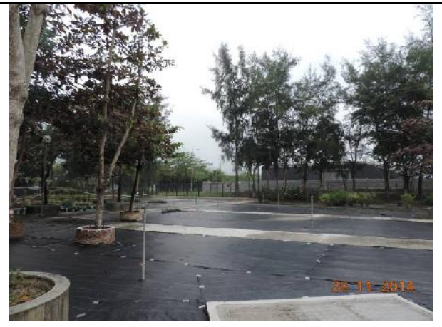
Photo 4 – The reinstatement work of the nursery ground in Phase 2 of Area B was completed.
