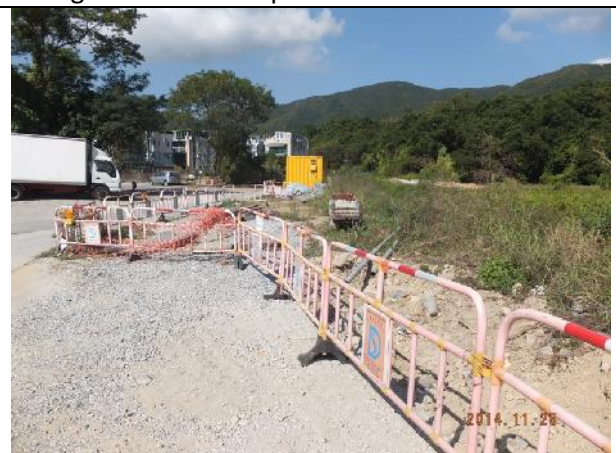
Photo 6 – Minor civil work was continued along the access path leading from Tung Tsz Road to Treasure Spot Garden II.
