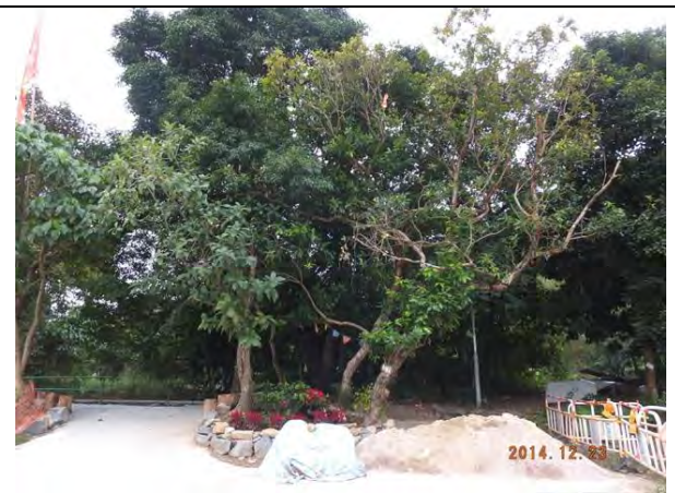
Photo 26 – Excavation work was noted very close to the tree group T181-T183 in May 2014. These trees have been surrounded by some stones to demarcate the tree group area by the villagers.
