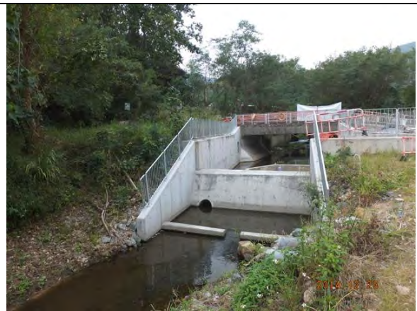
Photo 4 – Close-up view of the built drainage structure opposite to Wai Ha.
