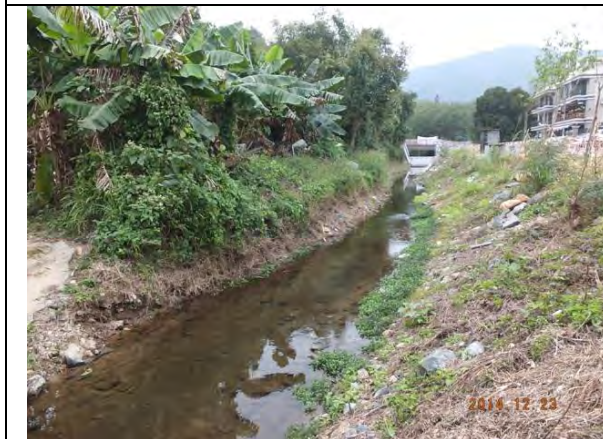
Photo 3 – All construction works along Wai Ha River were completed.
