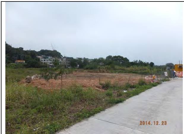
Photo 13 – A fenced area has been seen on the field next to the construction site along the access to Treasure Spot Garden II since March 2014.
