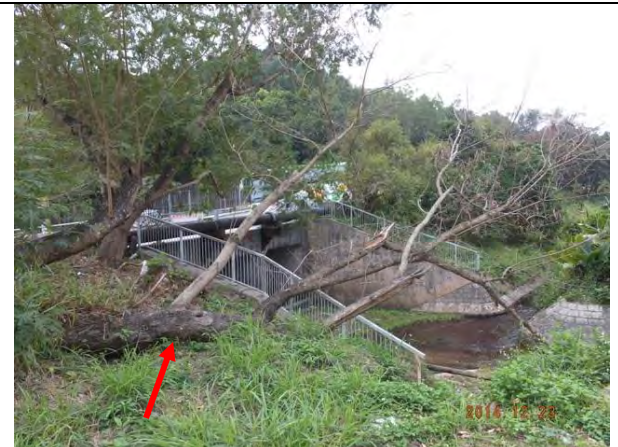
Photo 28 – The uprooted tree trunk leaned severely towards Wai Ha River.
