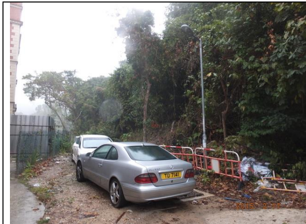
Photo 13 – Construction work at the end of the access path in Treasure Spot Garden II was finished. The works area was parked with villagers’ cars.
