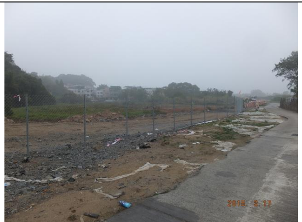
Photo 14 - A fenced area, which was erected by the villagers, has been recorded next to the works area of this Project.
