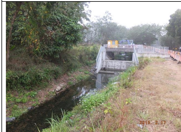
Photo 17 – The river water was clear as observed on 17 th February 2015.
