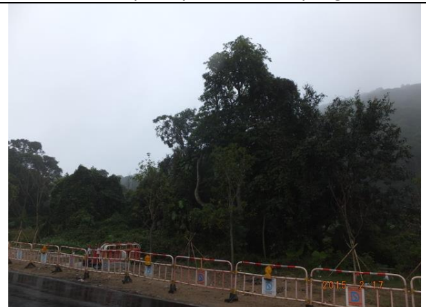
Photo 6 – Construction work opposite to Wai Ha area was already completed.
