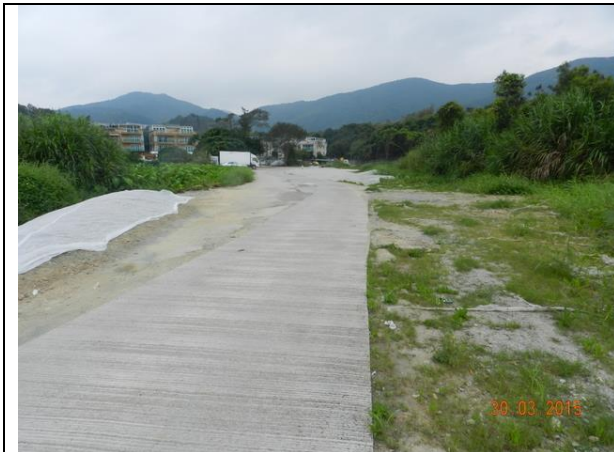
Photo B1 – Temporary hoardings along the access path towards Treasure Spot Garden II were removed.
