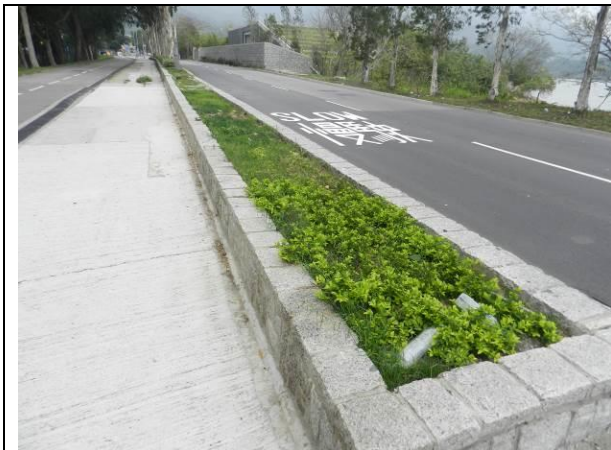
Photo A1 – Planters at Ting Kok Road were hydroseeded and planted with shrubs.
