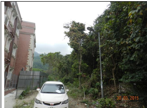
Photo B13 – Construction work at the end of the access path in Treasure Spot Garden II was finished. The works area was parked with villagers’ cars.
