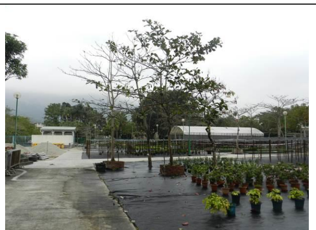
Photo A6 – Example of the completed reinstatement works within the nursery (such as lamp posts, shelters for potted plants and new planters for the transplanted tree).
