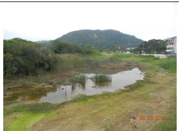
Photo B4 – Construction works opposite to San Tau Kok was already completed and fully vegetated.
