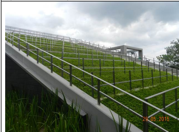
Photo A3 – View of sloping area with ground cover in the pump house.
