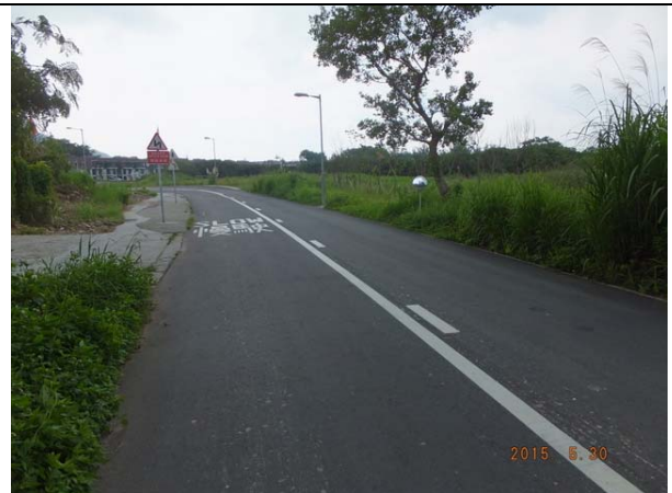
Photo B14 – The original access road (e.g. Tung Tsz Road) was reinstated.
