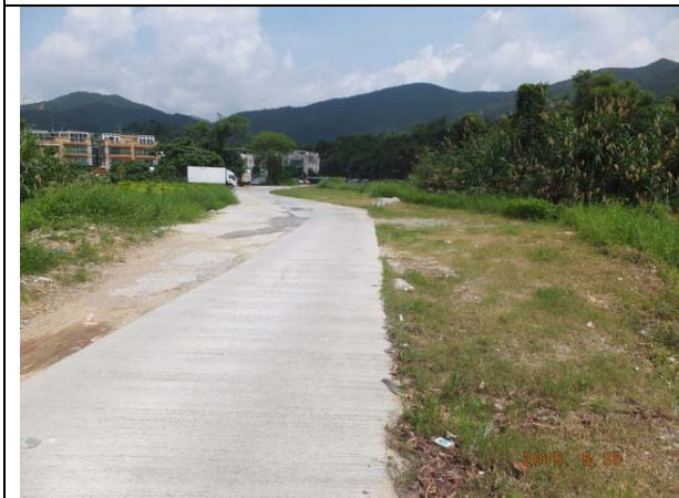
Photo B15 – The access path leading to Treasure Spot Garden II was reinstated.
