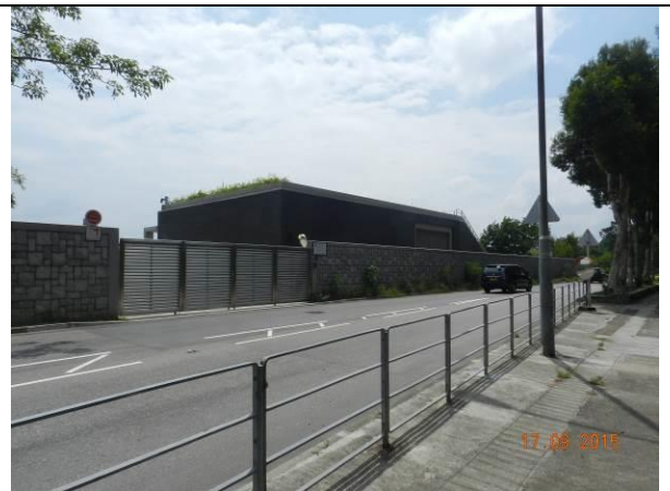
Photo A2 – General appearance of the pump house in Area A.
