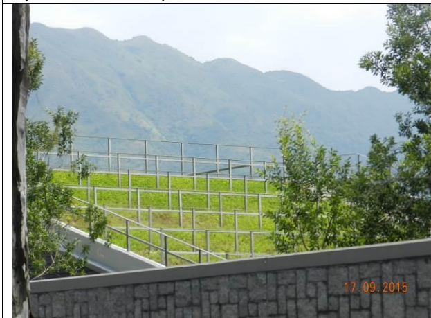
Photo A3 – View of sloping area with ground cover on the Pump House.
