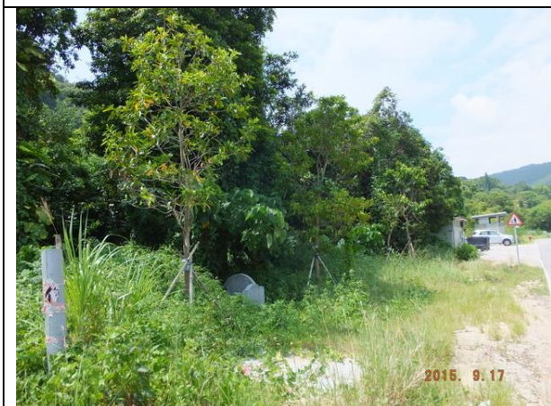
Photo B9 – Hydroseeding was applied on the reinstated soil ground above the alignment of the box-culvert along Tung Tsz Road.
