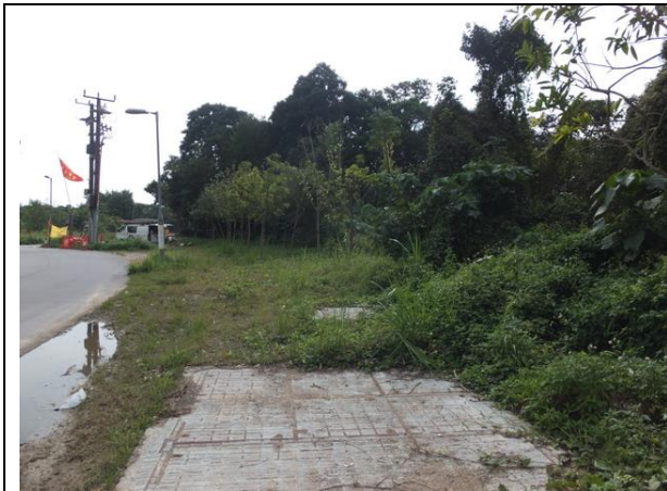
Photo B7 – Hydroseeding was applied on the reinstated ground above the alignment of the box-culvert along Tung Tsz Road.
