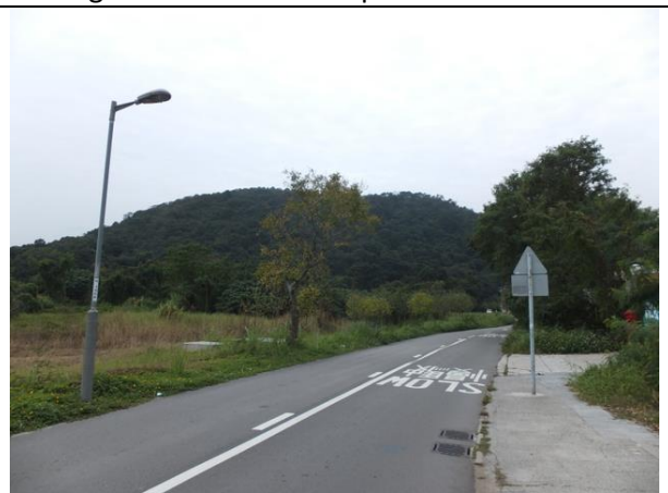
Photo B10 – The original access road, Tung Tsz Road, was reinstated.
