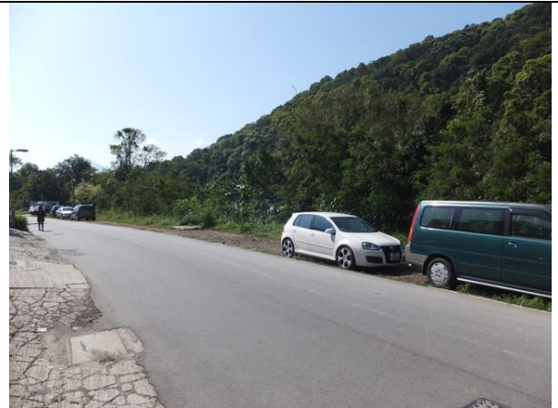
Photo 20 – The original access road, Tung Tsz Road, was reinstated.
