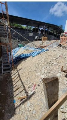
1. The exposed soil surface was covered with impervious sheeting. to mitigate construction dust pollution
