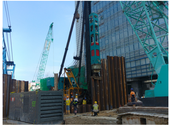
Site inspection photo of 11 th May 2017
