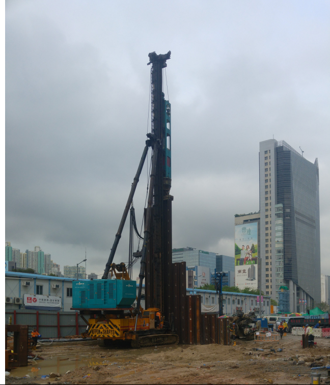
Site inspection photo of 4 th May 2017
