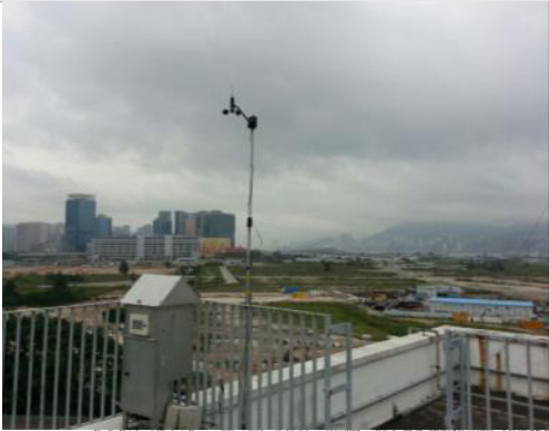
Wind Data Monitoring Equipment set at Lee Kau Yan Memorial School
