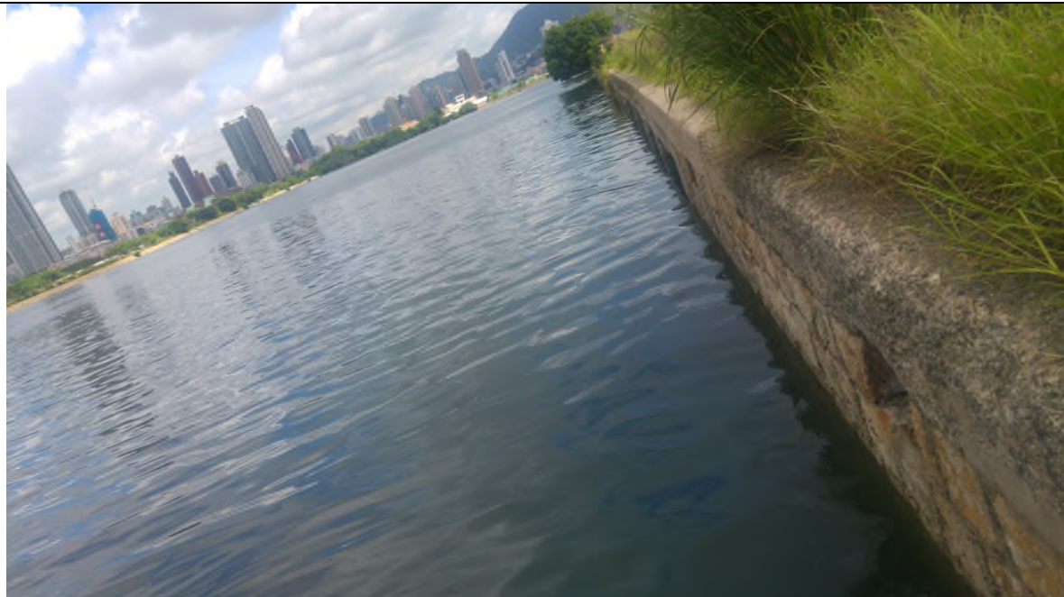
Existing 7-cell box culvert outfall
