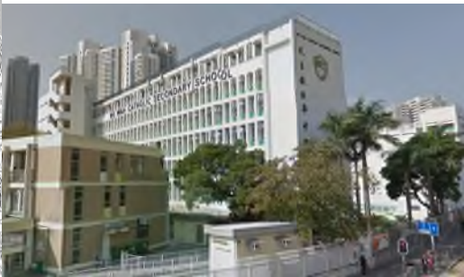
Wind Data Monitoring Equipment set at AM2(A) - Ng Wah Catholic Secondary School
