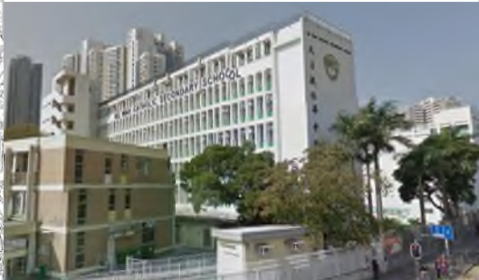
Wind Data Monitoring Equipment set at AM2(A) - Ng Wah Catholic Secondary School
