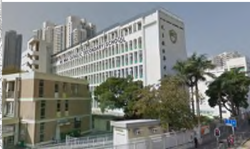
Wind Data Monitoring Equipment set at AM2(A) - Ng Wah Catholic Secondary School
