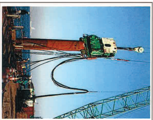
Piling, vibrating hammer 打樁機，震動錘
