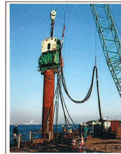
Piling, vibrating hammer
