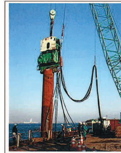
Piling, vibrating hammer 打樁機，震動錘
