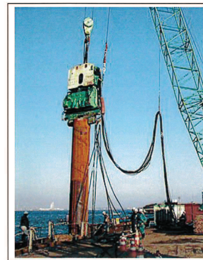
Piling, vibrating hammer 打樁機，震動鎚
