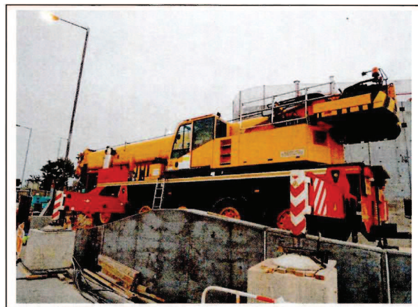
CNP 048 Crane, mobile (diesel) 起重機，流動 (油渣)
