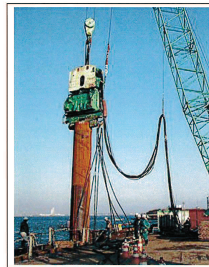
Piling, vibrating hammer 打樁機，震動錘
