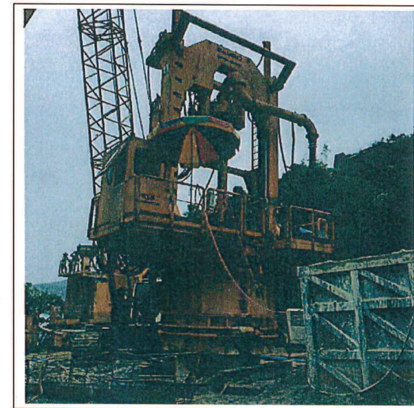
CNP 166 Piling, large diameter bored, reverse circulation drill 大直徑鑽孔樁，循環式鑽機
