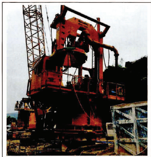
CNP 166 Piling, large diameter bored, reverse circulation drill 大直徑鑽孔樁，循環式鑽機
