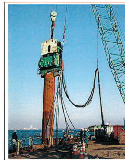
Piling, vibrating hammer 打樁機，震動錘
