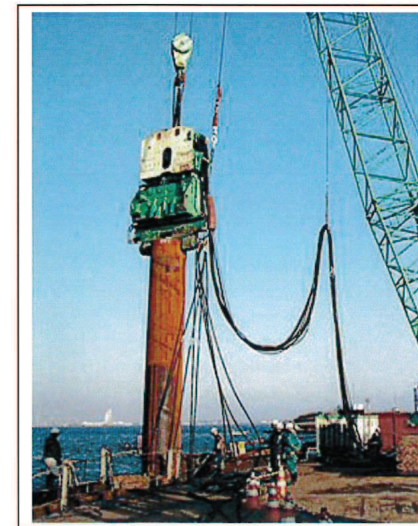
Piling, vibrating hammer
