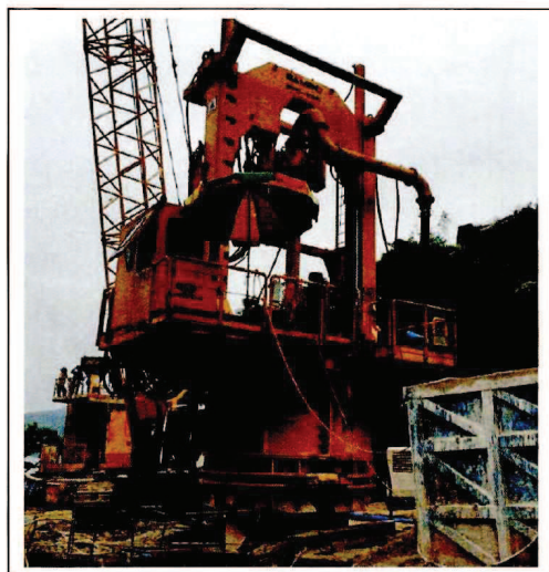
CNP 166 Piling, large diameter bored, reverse circulation drill 大直徑鑽孔樁，循環式鑽機
