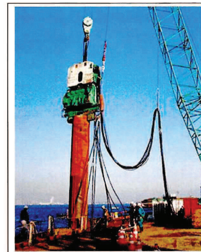
Piling, vibrating hammer 打樁機，震動錘
