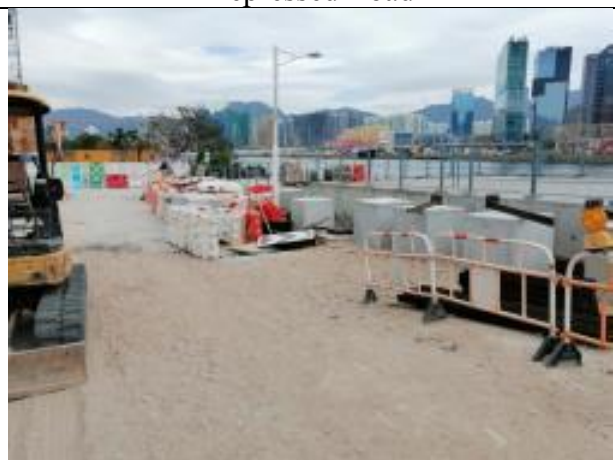
Construction of Hoarding
