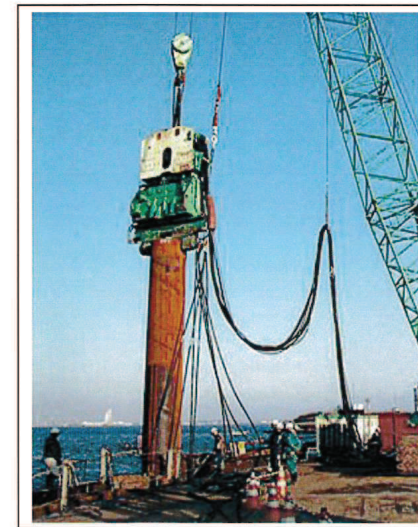
Piling, vibrating hammer 打樁機，震動鎚
