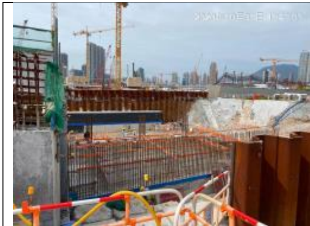
Construction of base slab, walls and columns for North Approach Ramp
