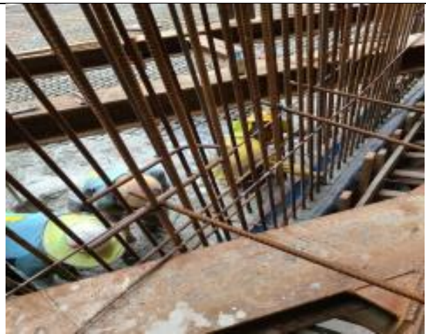
Permanent Structure Construction for North Depressed Road
