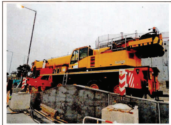
CNP 048 Crane, mobile (diesel) 起重機，流動 (油渣)
