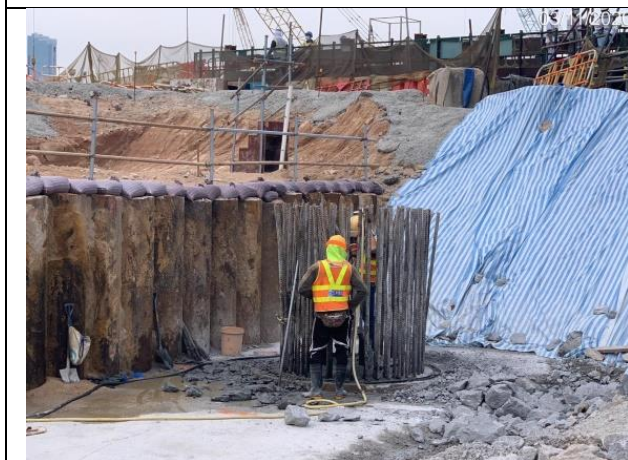
Permanent Structure Construction for Pile Cap of Bridge D3
