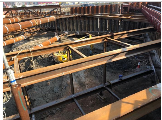
Excavation, pumping test and ELS for Underpass and South Depressed Road
