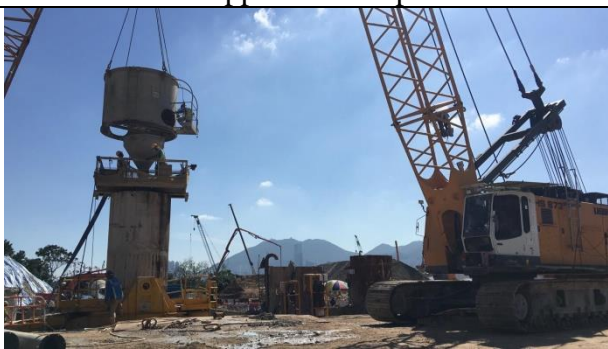
Bored Pile Construction for Bridge D3
