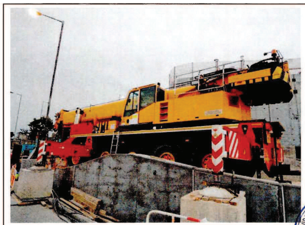
CNP 048 Crane, mobile (diesel) 起重機，流動 (油渣)
