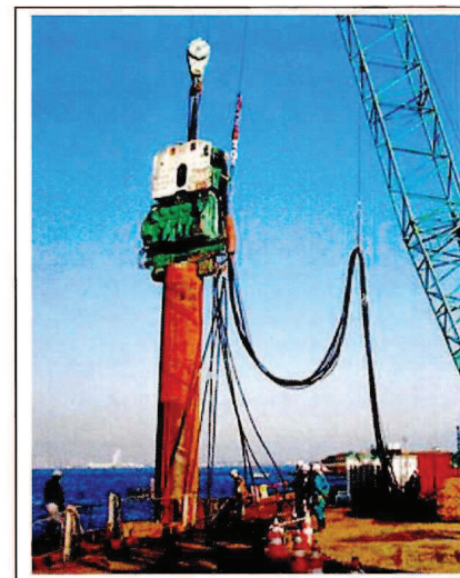
Piling, vibrating hammer 打樁機，震動錘
