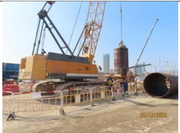
Elevated landscape deck – Bored Pile
