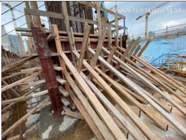
Construction of Permanent Structure for Pile Cap
