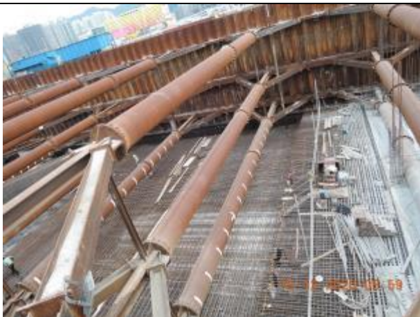
Excavation and ELS for Underpass and South Depressed Road
