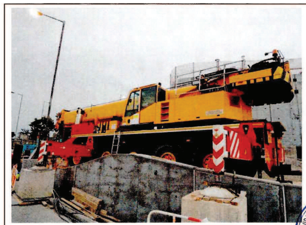
CNP 048 Crane, mobile (diesel) 起重機，流動 (油渣)
