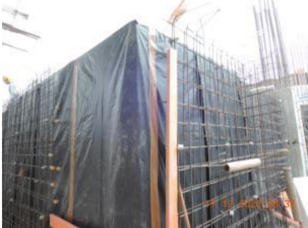
Construction of base slab and wall for North Approach Ramp
