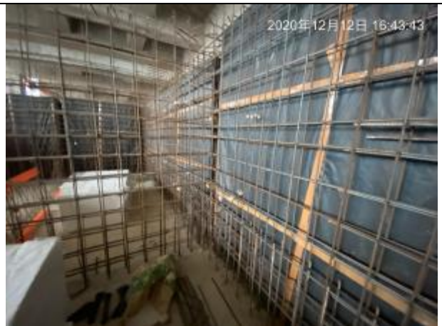
Metal Scaffolding and Falsework Erection & Dismantling at North Approach Ramp
