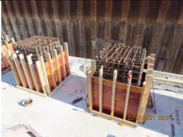
Noise barrier - Construction of footings
