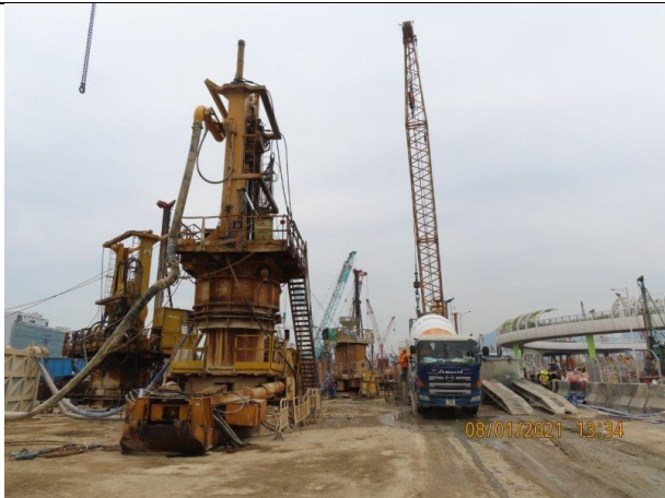
Landscaped Deck – Construction of bored piles
