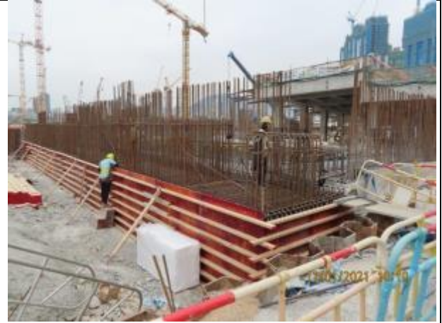
Bridge D3 – Construction of pile cap
