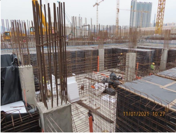
North Approach Ramp – Construction of wall, intermediate slab and column
