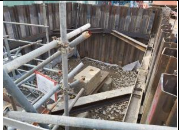
Lift 3 – Construction of cofferdam for footing
