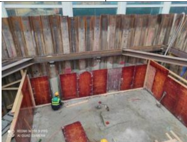
Lift 3 – Construction of cofferdam for footing
