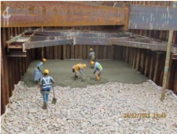
District Cooling System seawater intake box culvert - Construction of cofferdam
