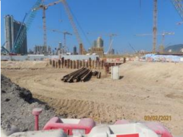
South Approach Ramp – Installation of sheet pile and excavation
