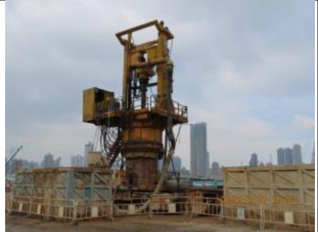
Landscaped Deck – Construction of bored piles
