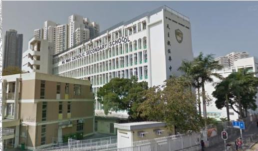
Wind Data Monitoring Equipment set at AM2(A) - Ng Wah Catholic Secondary School
