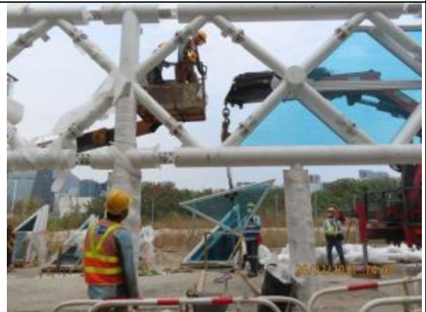
Noise barrier – Installation of steel structure and PMMA panel
