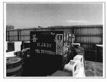
Generator, with Quality Powered Mechanical Equipment Label showing a Sound Power Level ≤93 dB(A) (1) 發電機,備有優質機動設備標籤顯示聲功率級≤93 分貝(A) (一)
