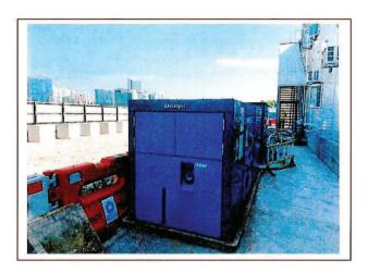
Generator, with Quality Powered Mechanical Equipment Label showing a Sound Power Level ≤93 dB(A)
