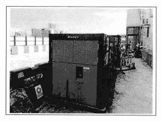
Generator, with Quality Powered Mechanical Equipment Label showing a Sound Power Level  $\leq$  93 dB(A)
