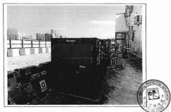
Generator, with Quality Powered Mechanical Equipment Label showing a Sound Power Level ≦93 dB(A) (2) 發電機,備有優質機動設備標籤顯示聲功率級≦93 分貝(A) (二)
