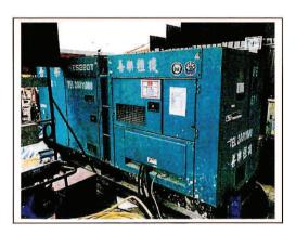
Generator, with Quality Powered Mechanical Equipment Label showing a Sound Power Level of ≤94 dB(A) 發電機,備有優質機動設備標籤顯示聲功率級≤94分貝(A)
