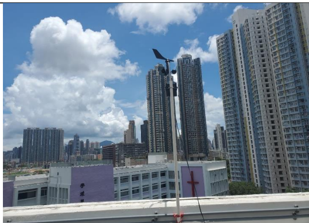
Weather Station at the rooftop of Ng Wah Catholic Secondary School
