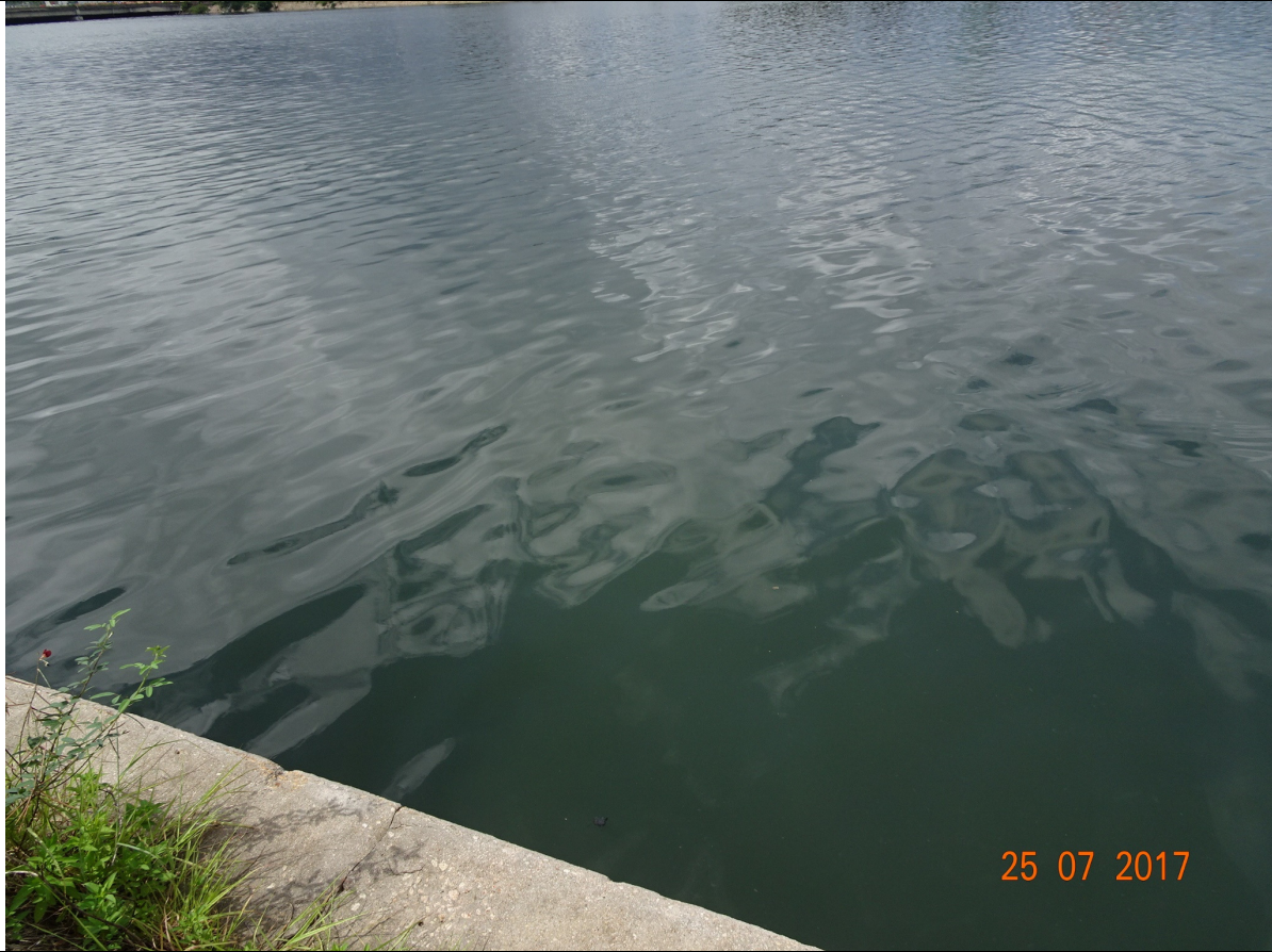
Dye traced at the 7-cell box culvert outfall
