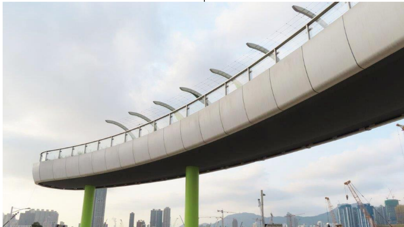
Reference photo of Elevated Landscaped Deck structure located at Kai Tak Stage 2 Development, form of deck structure, color and surface details to be echo and incorporated in this contract.
