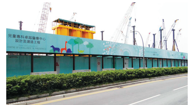
Figure 6 Centre of Excellence in Paediatrics Construction Site Hoarding
