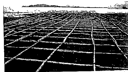
Mirafi® woven geotextile used as a basal filter in breakwater construction
