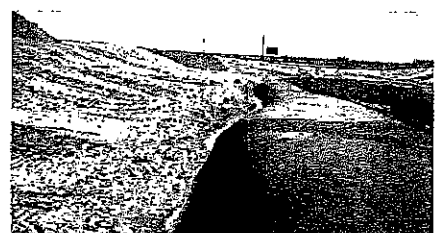
Mirafi® woven geotextile used to construct capping layer over very soft tailings
