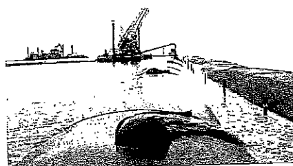
Geotube® containment units used to construct dykes for land reclamation
