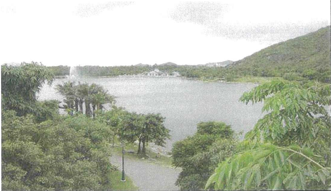
Inspiration Lake with HDPE geomembrane waterproofing system, Disneyland Hong Kong, 2005
