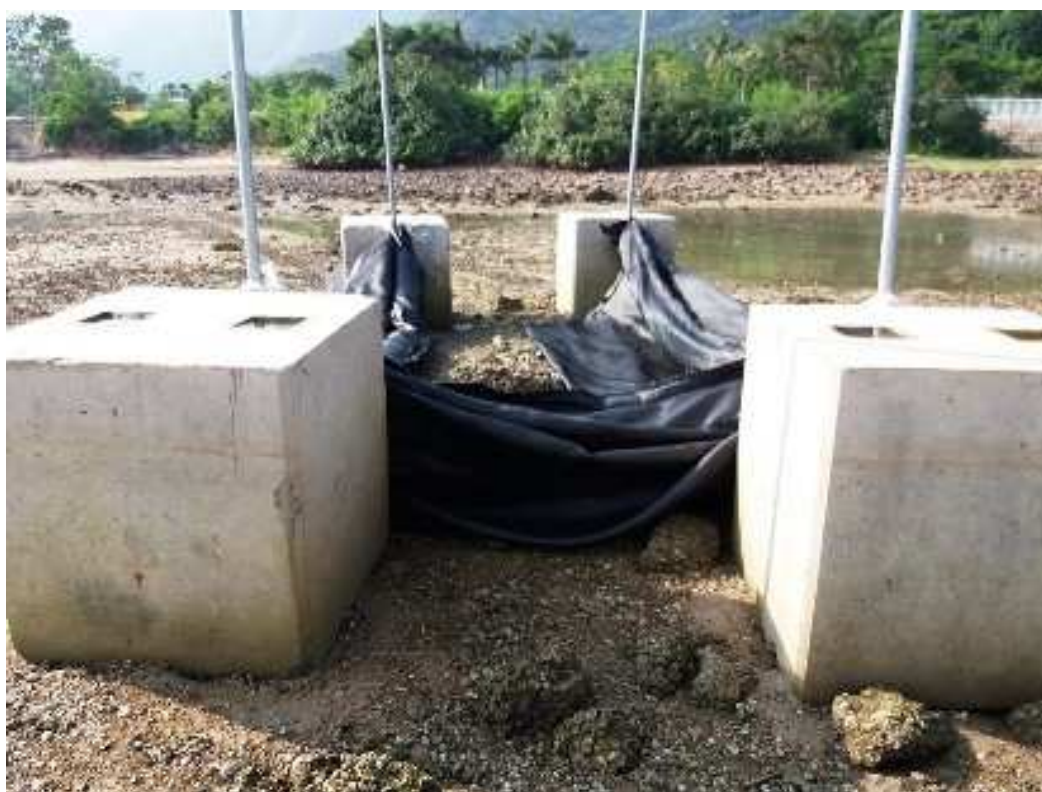
Photo 1. Close-up of the fencing structure with concrete blocks and silt curtain
