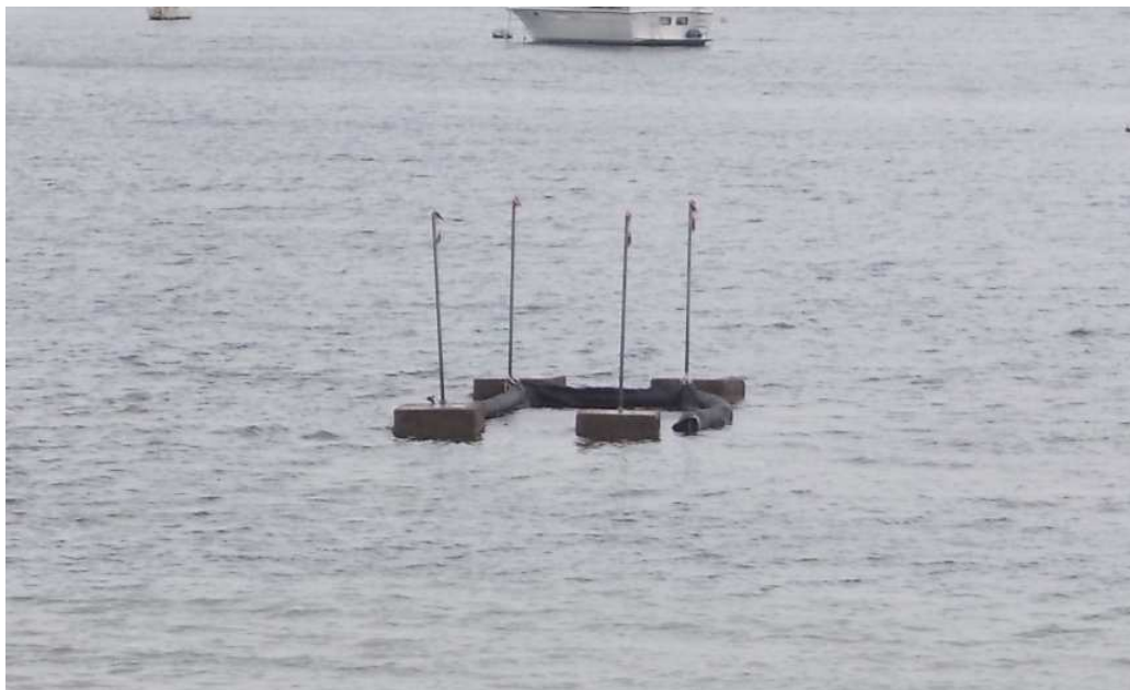
Photo 3. Demonstration of the fencing structure with concrete blocks and silt curtain in water
