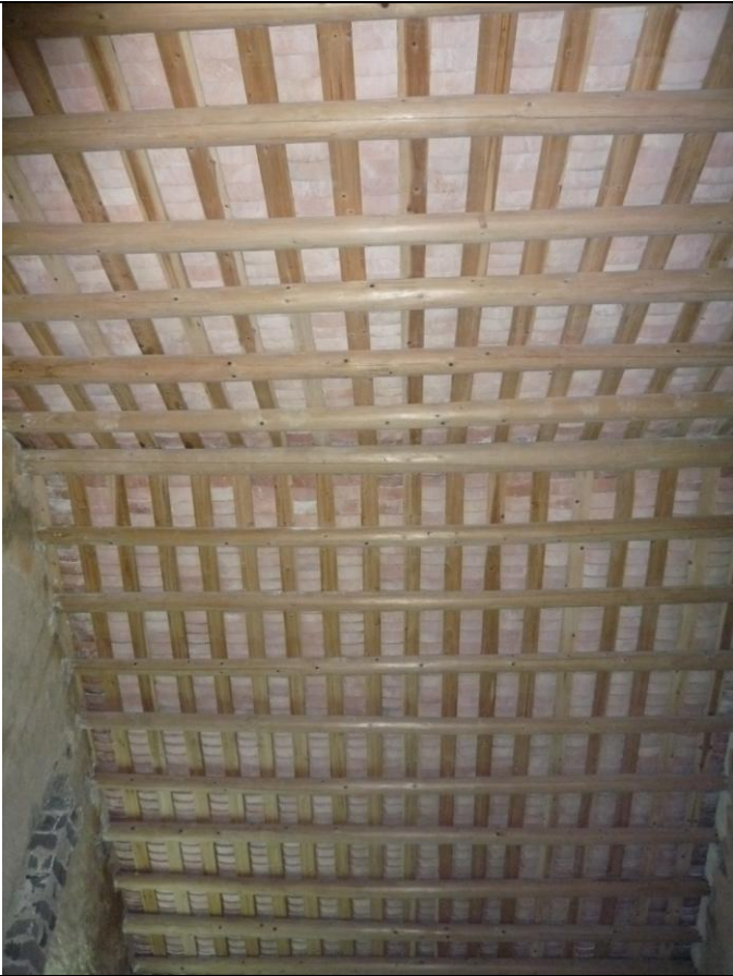
Kitchen Annex – Roof (30/8)
