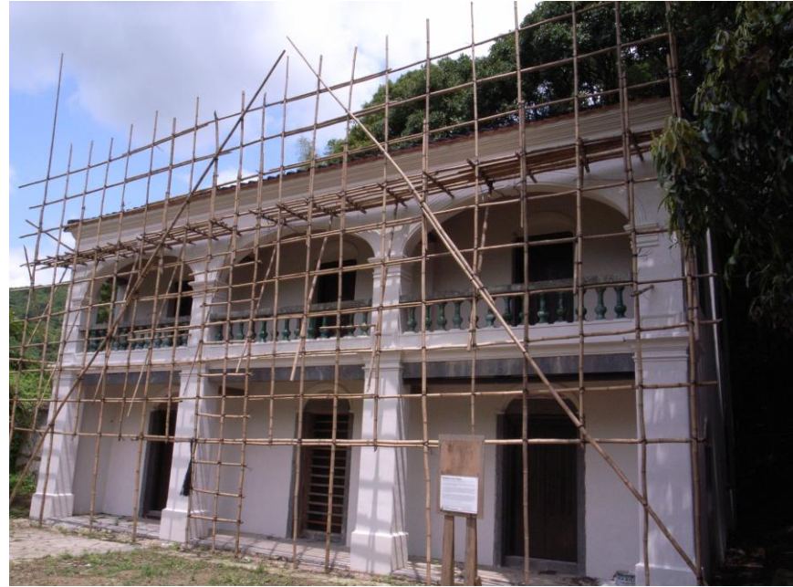
Scaffolding at Main Building (14/7)
