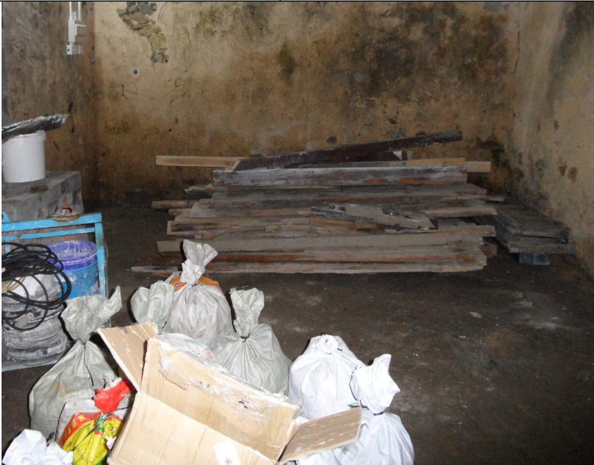
Kitchen Annex – Floor (15/8)
