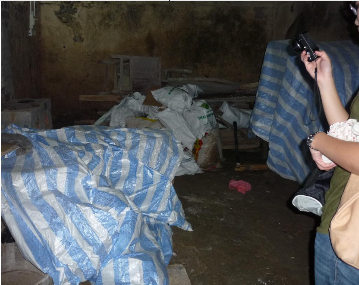
Kitchen Annex – Floor (30/8)
