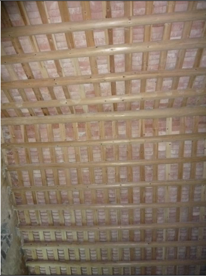
Kitchen Annex - Roof (15/8)
