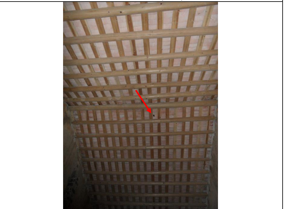
Kitchen Annex - Roof (27/9)
