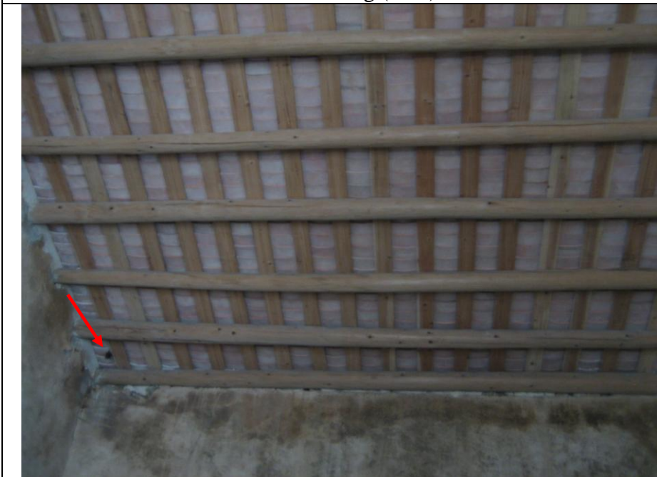
Kitchen Annex - Roof (15/9)
