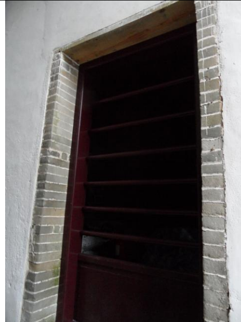
Kitchen Annex – Bat Gate (27/9)
