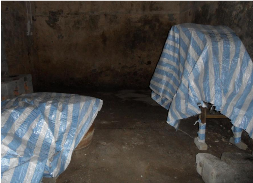
Kitchen Annex - Floor (27/9)
