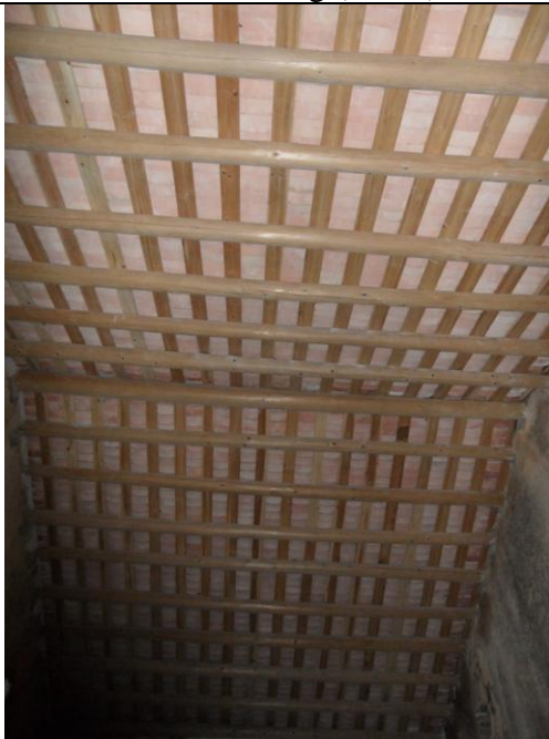
Kitchen Annex - Roof (27/10)
