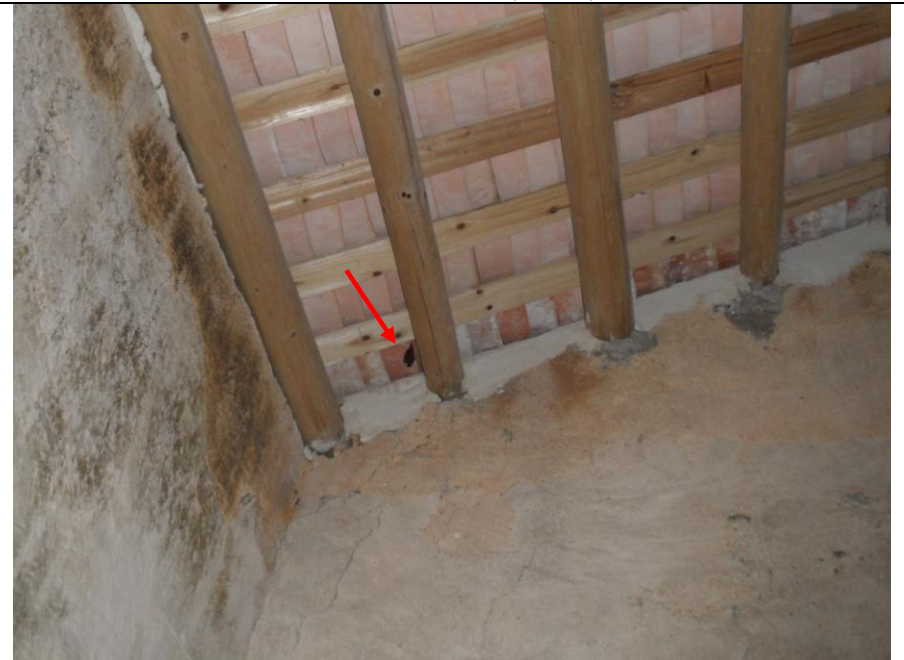
Kitchen Annex - Roof (27/10)
