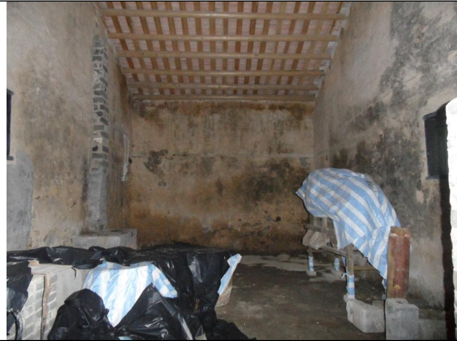
Kitchen Annex - Floor (01/11)
