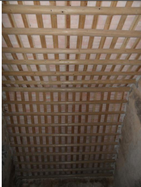
Kitchen Annex - Roof (01/11)
