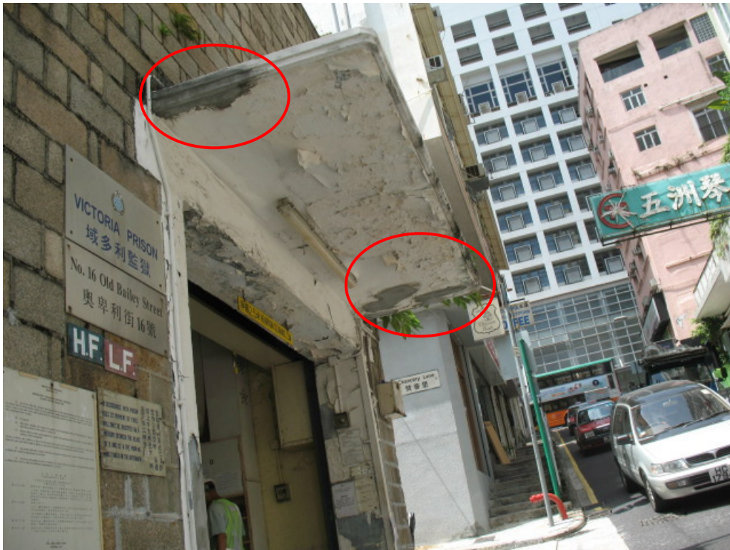
Photo ex 23a – The canopy is repaired.
