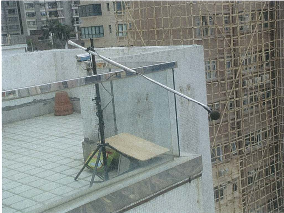
Alternative Baseline Noise Monitoring Station (N6)
