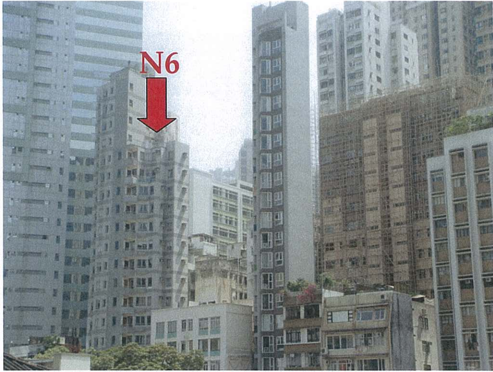
Alternative Baseline Noise Monitoring Station (N6)
