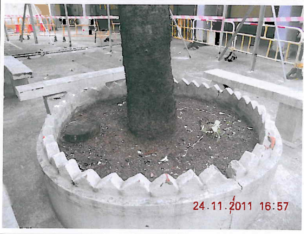
Fig. 3 Under-growth and rubbish have been cleared prior to inspection, The planter keeps clean and tidy.
