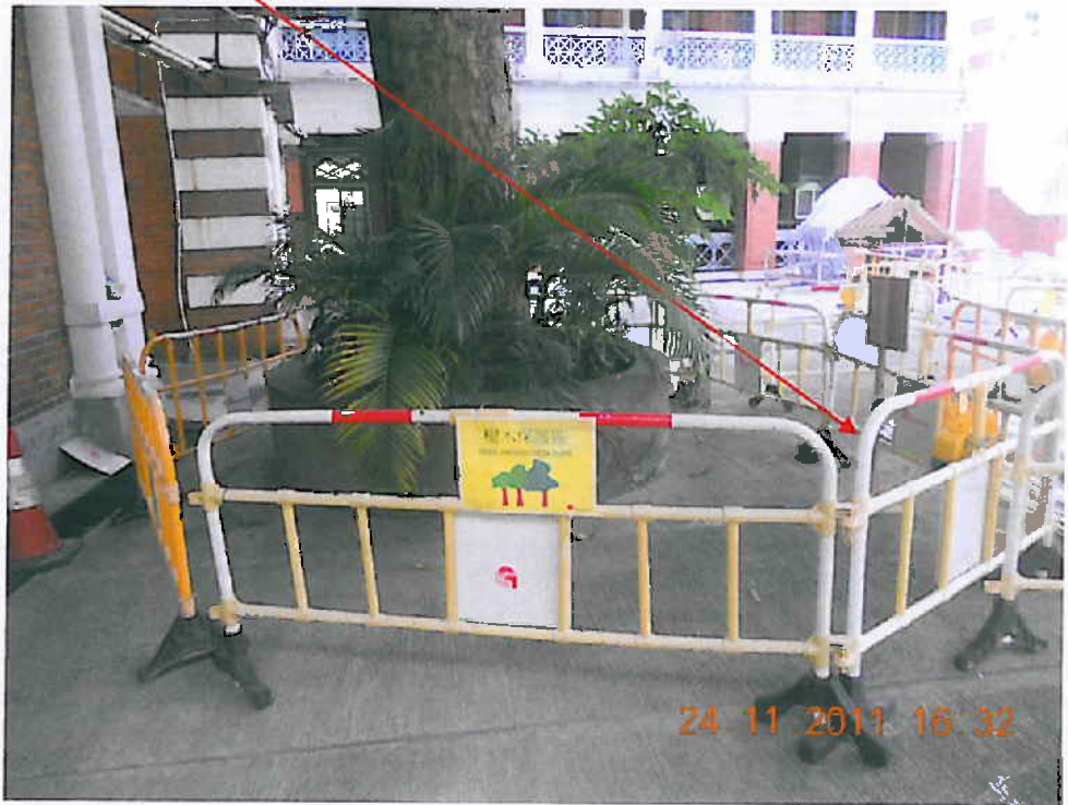
Fig. 4 The rails have been linked up as a temperate protection zone.
