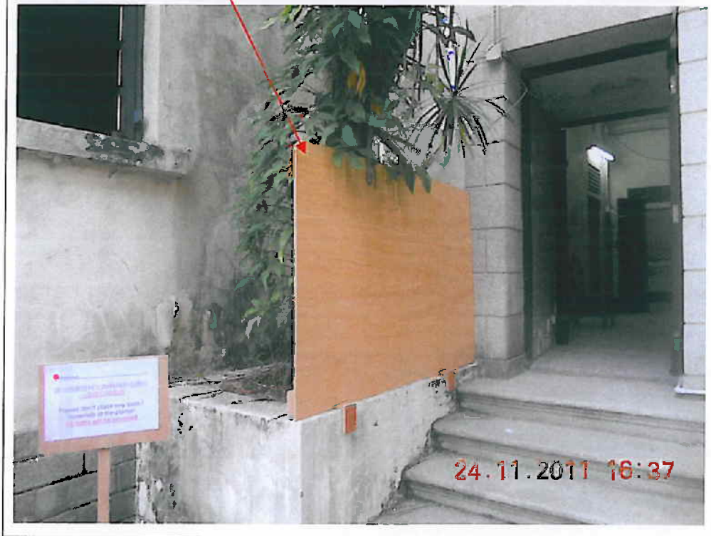
Fig. 4 Temperate fence has been erected at the planter.
